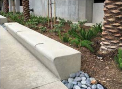
Concrete Seatwall (18" Ht.)
